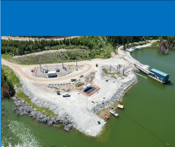
Overhead view in situ application infrastructure
